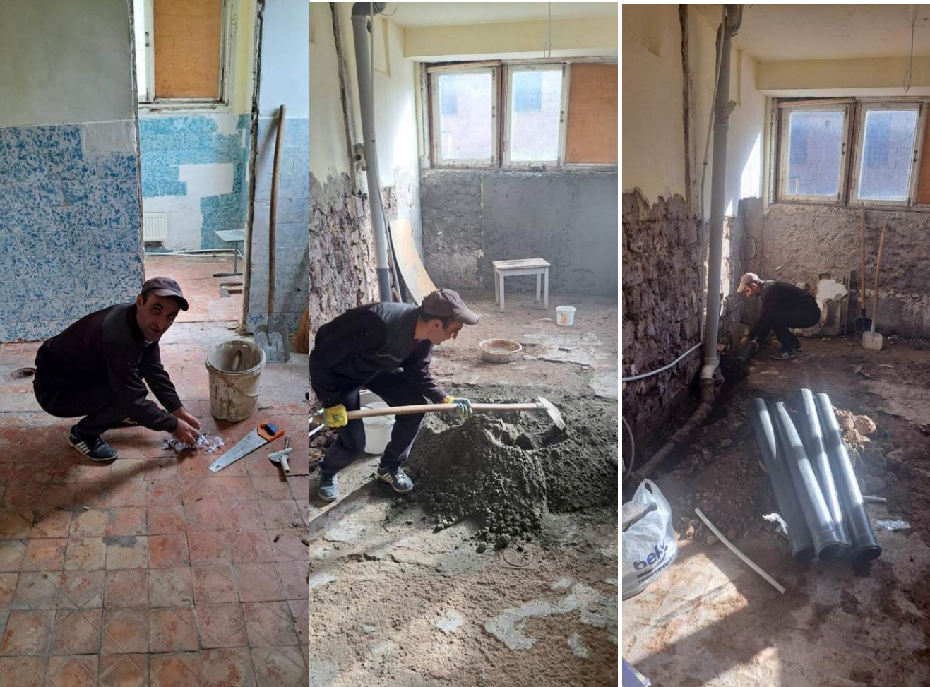
Demolition of the old toilet
