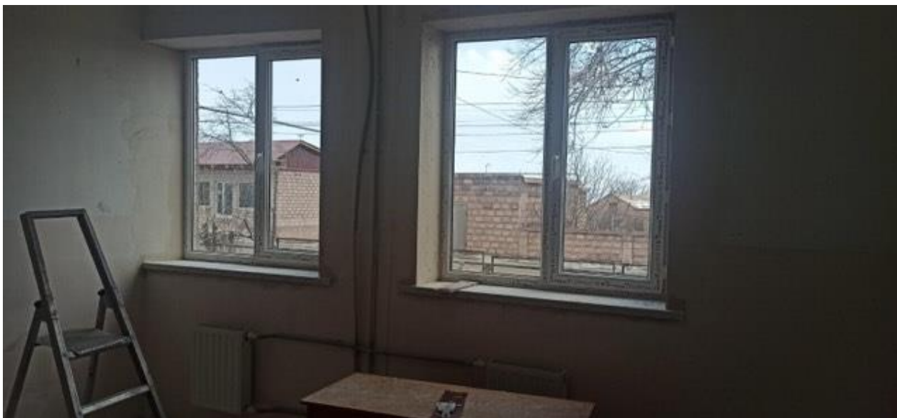
Newly installed windows
