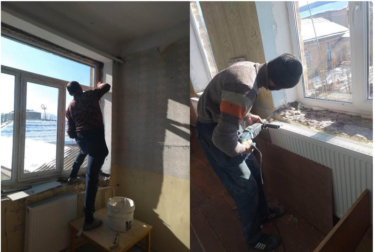
Installation of new windows, doors and window sills
