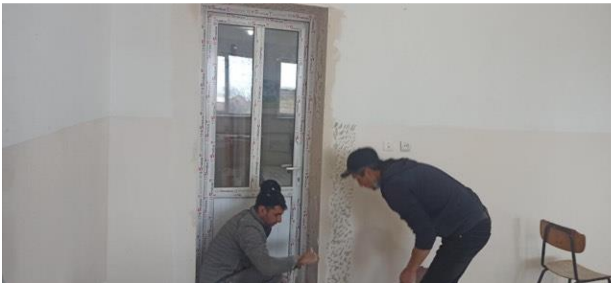
Interior finishing works
